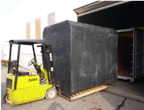
Installation of the bio module in a sea container
