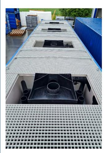
The ClearFox® DAF is a fully automated unit. The wastewater to be treated is fed from the customer's surge tanks or ClearFox® buffer tanks to the DAF via a non-clogging cavity pump. The use of aerated buffers is recommended for certain applications.
