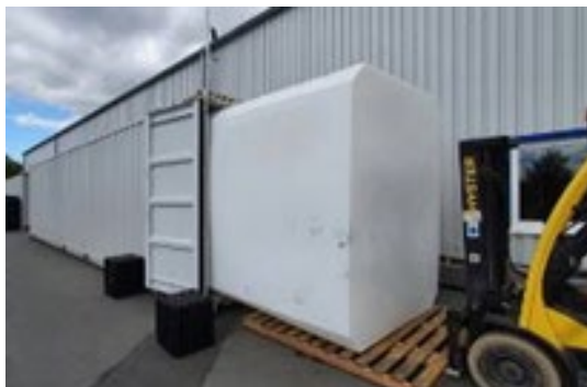
buffer installation into a sea container
