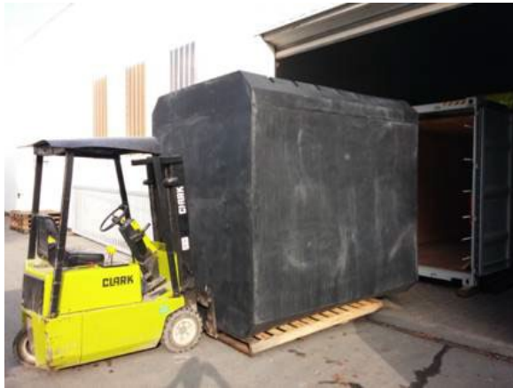
Installation of the bio module in a sea container
