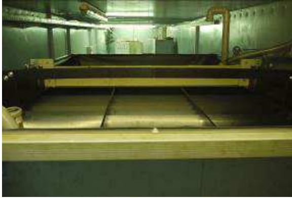
Internal view machine container
