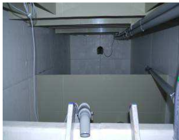
sludge treatment, Emscher, secondary sludge removal installation, 450 p.e treatment system
