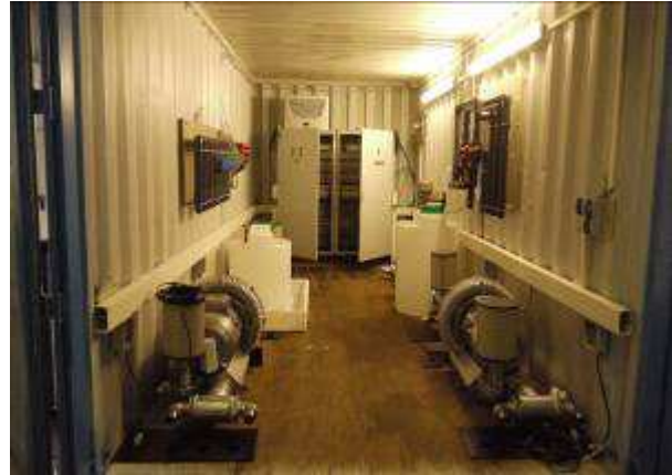
view inside machine house, non frost protected container, 3.000 p.e
