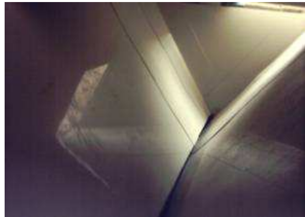
view into settling zone (Emscher)
