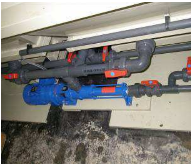
secondary sludge pump (excentric pump), line from lamella clarifier to sludge storage
