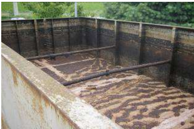
open top sludge container&aeration,stabalizing
