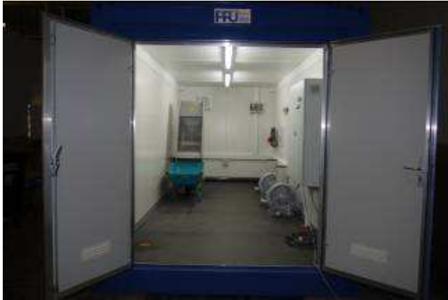
view inside , machine house , frost protected container, 1000 p.e
