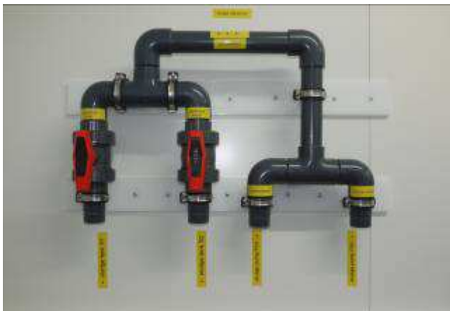
sludge splitter into storage tanks, labeling in english language
