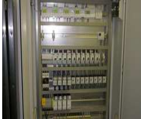
Control unit with modem for failure transfer to mobile phone (SMS per GSM), free programmable
