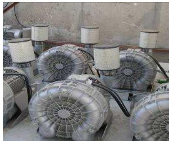
blow er battery extended 500 m 3 /d mixed water
