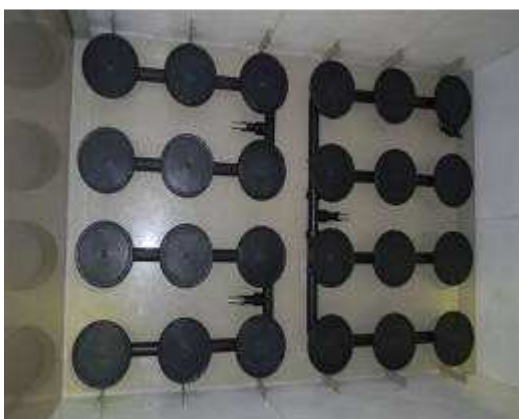
1 cascade – aeration and mixing system in 1 .cascade
