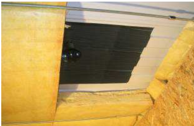
Insulation in container 120 mm thickness, roof view
