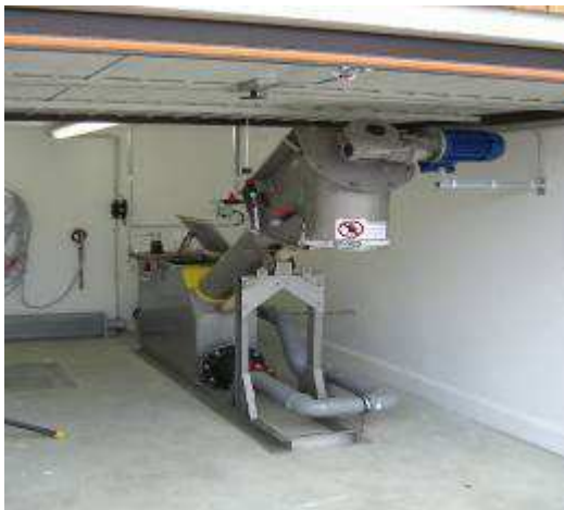
screw screen with bypass
