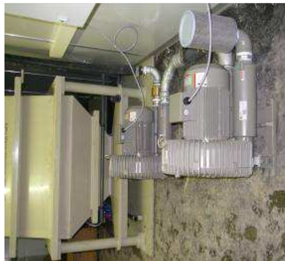
sludge hoppers in lamellar clarifieer (back) small blowers for buffer preaeration & mixing (front)
