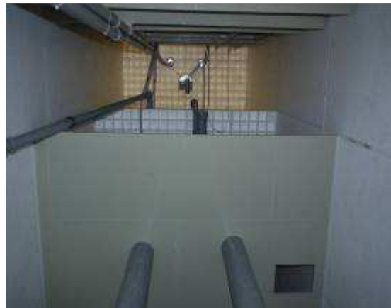
baffles and tubes inside the 20 ft inlet
