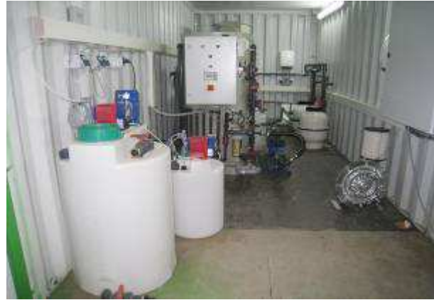
precipitation and UV treatment, 2.500 people equivalent non insulated 20 feet container
