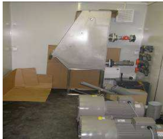
machine house: mechanical screen, blowers sludge splitter
