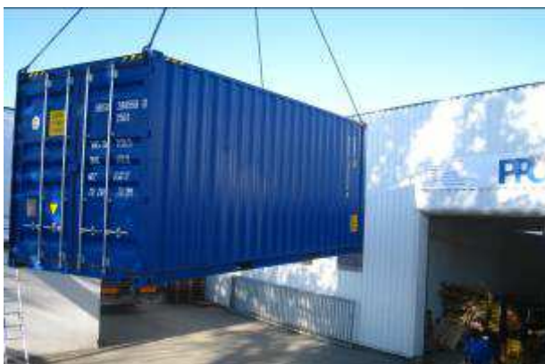
lifting a Container in High Cube 20 ft out of production hall inside a fixed bed cascade 850 person equivalent
