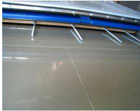
Reinforcements & tie bars along side walls, fixed bed
