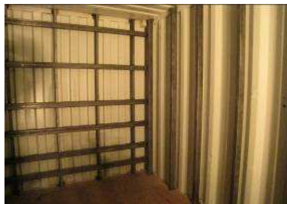
Reinforcement inside fixed bed container with steel profiles according to a static approval of a german design specialist
