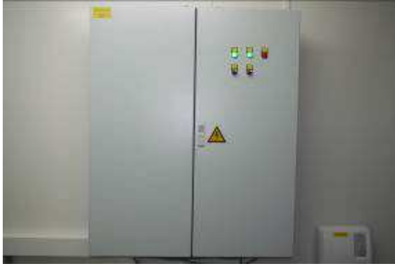
Control cabinet outside
